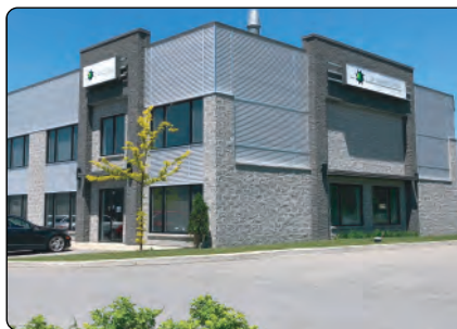
Solaris R&D Synthetic Laboratory Facilities, Vaudreuil-Dorion, Quebec, Canada
